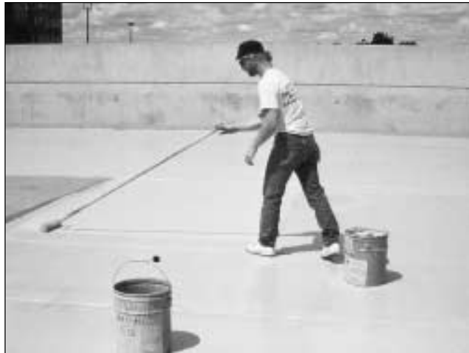
Roller cover application of the intermediate coat.
